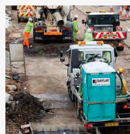
Mains and waste connected
