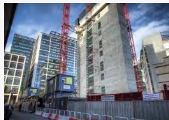
Can be cited under kitchens, canteens, toilet blocks and welfare units
