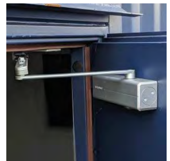
Door Closers Door closers fitted to all external doors.
