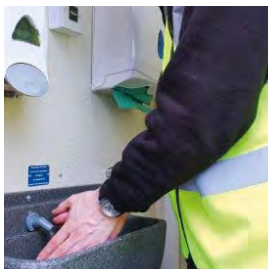
Delivery of hot water Warm water is delivered instantaneously via a 12V pump.
