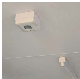
PIR Sensors Energy efficient PIR sensors only turn the lights on when the unit is in use, automatically switching off when no motion is detected.
