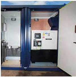
9.8KVA diesel generator Diesel generator to power the unit.
